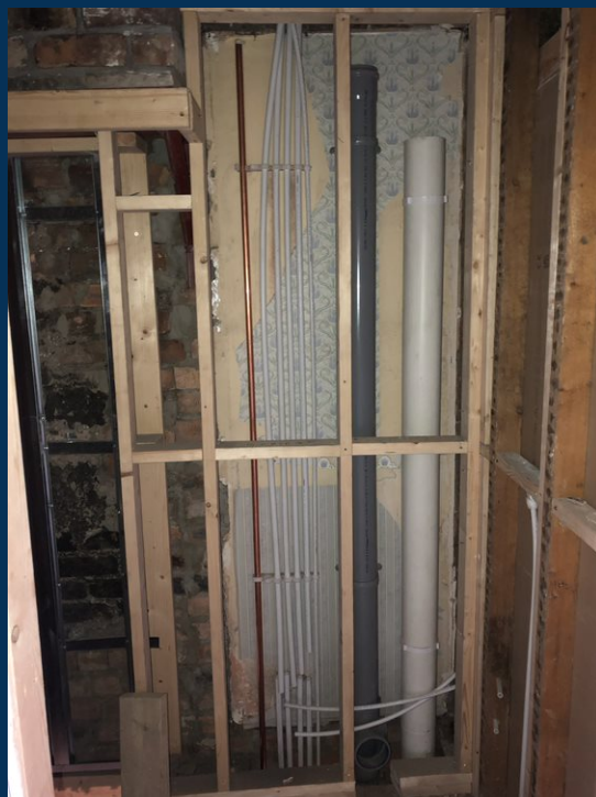
First fix pipe work
